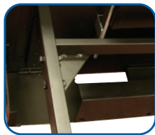
Stretcher Bar & Corner Braces
